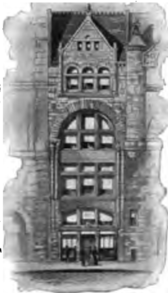
COLLEGE BUILDING 202 MICHIGAN BOULEVARD
