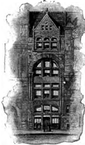
COLLEGE BUILDING 202 MICHIGAN BOULEVARD
